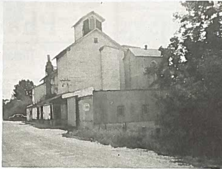
THE HOLMES MILLING COMPANY MILL --In the late 1950s or early 1960s. The mill had gone off water power and had taken on electricity to run the grinding machines, but it still put out only animal feed and custom grinding. The famed Log House pancake flour and the Klondike bread flour had long since been discontinued. From an old photo.
