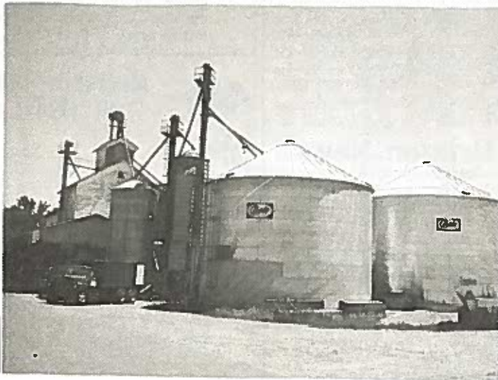
THE SAME MILL TODAY --Under Bader Milling Company ownership. Shown above are two of the three huge grain storage tanks Bader's have built (the third is aligned behind one in the foreground, in the photo). Each storage bin can hold 22,000 bushels of wheat or corn. The first big storage bin was built three years ago by Bader's, then one last year, and the third was recently completed. Messenger photo
