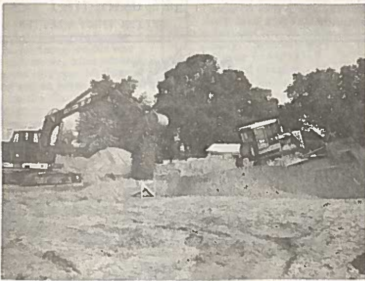
EXCAVATIONS FOR THE NEW BANK BUILDING --Are deep and extensive. An area dug for the full basement of the new building was down over 10 feet last weekend. This of course will be partly filled in after tile, water and electric lines have been installed.
